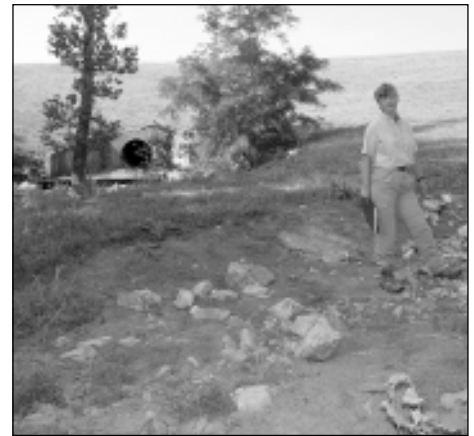
TOP and LOWER RIGHT: Dam safety inspector Marilyn Thomas checks the downstream embankment of Pulliam Dam for slumps and slides that could be symptomatic of seepage. ABOVE LEFT: Thomas checks for debris and other obstructions on the trash rack covering the principal spillway on Pulliam Dam. CENTER: Thomas evaluates the condition of the drawdown valve at Pulliam Dam. Photos by Allison Fleck
