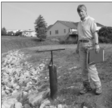
TOP and LOWER RIGHT: Dam safety inspector Marilyn Thomas checks the downstream embankment of Pulliam Dam for slumps and slides that could be symptomatic of seepage. ABOVE LEFT: Thomas checks for debris and other obstructions on the trash rack covering the principal spillway on Pulliam Dam. CENTER: Thomas evaluates the condition of the drawdown valve at Pulliam Dam. Photos by Allison Fleck
